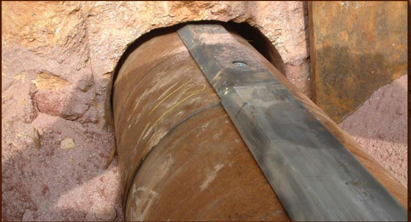
*The Front Steer Guided Auger Boring system can excavate extremely hard ground up to 100 blow counts/12" or up to 2,900 psi soils and as small as 16" in diameter.*
